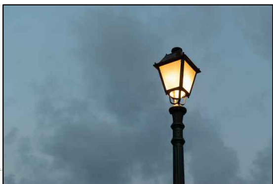
TYPICAL STREET/SIDEWALK LIGHT W/ FIBERGLASS POLE
