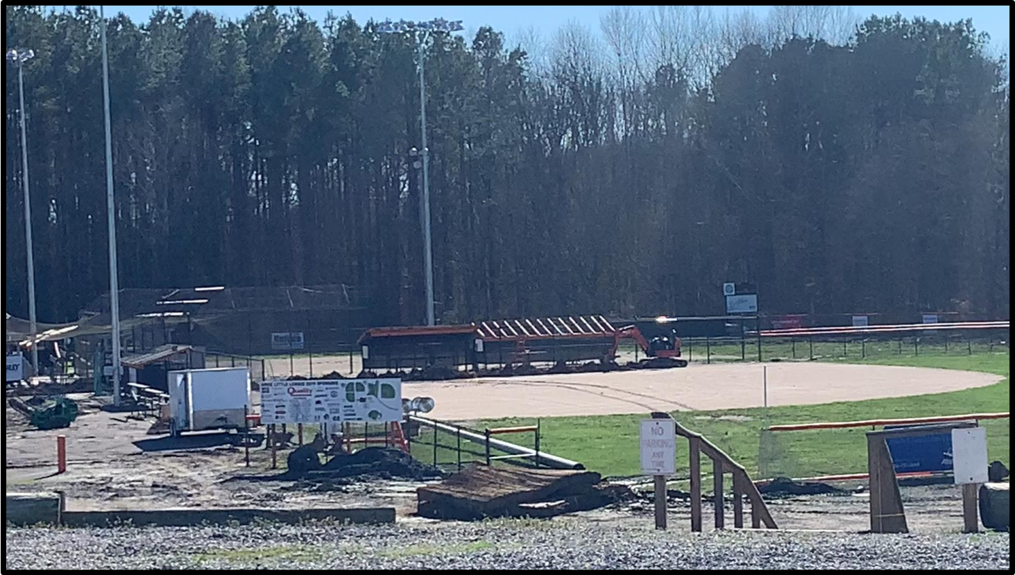
Blasting for new lights
