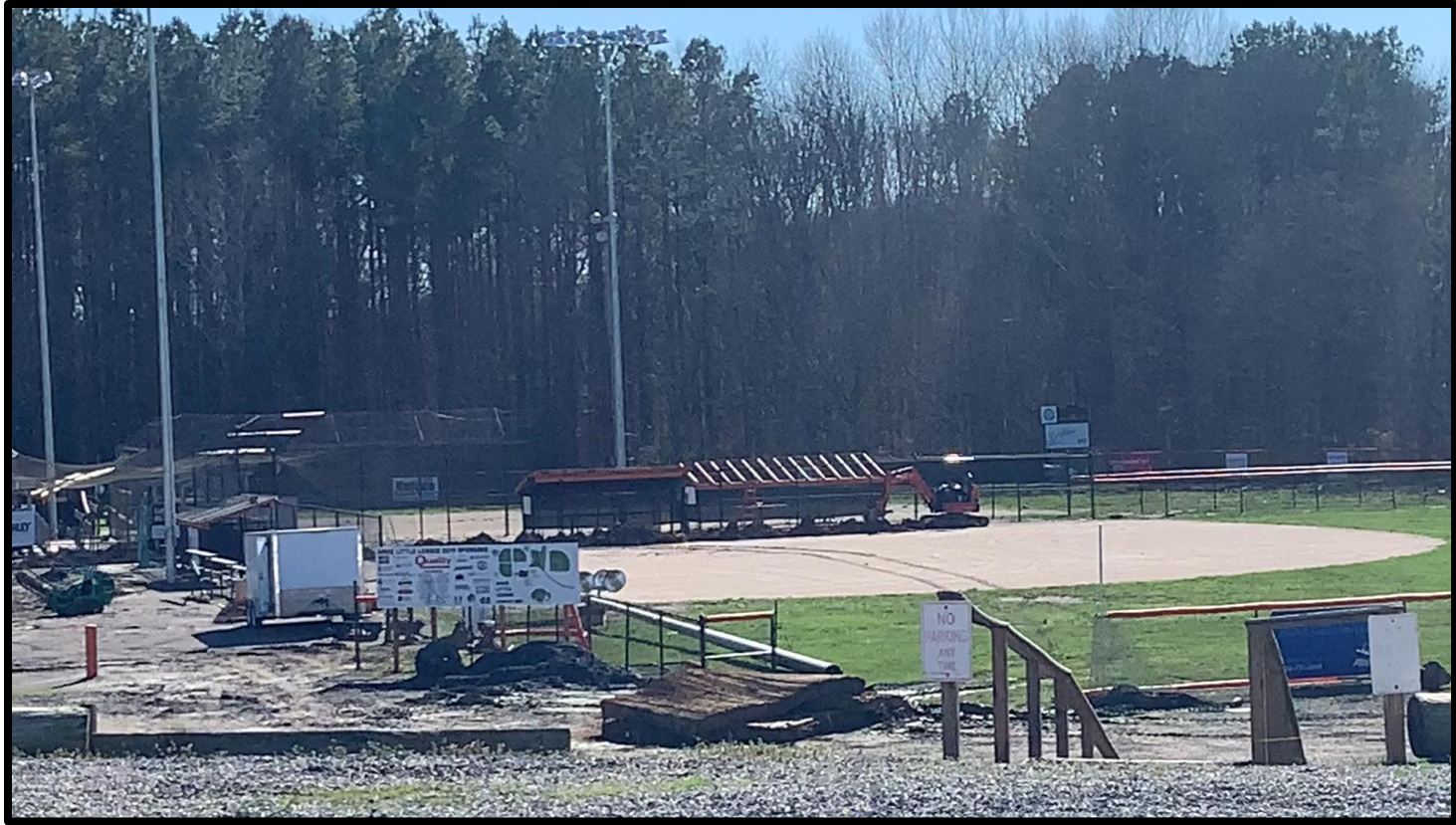
Blasting for new lights
